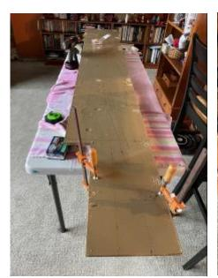
Virgin (almost) plywood tabletop! This is the first or southern section of Kingfield. Pressure treated 2x4's are clamped to the plywood. They are screwed together using exterior grade deck screws.
