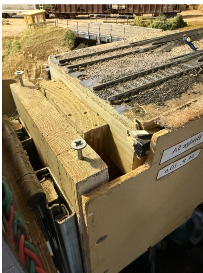
A closeup of the abutment on the helix with Bridge 5 'down'. From left to right: lever switches for the kill sections, adjustment screws to maintain proper cross level, ends of the two drawer slides that allow the bridge to lift and finally the pivot of the door hinge attached to the slides that allows the bridge to pivot.
