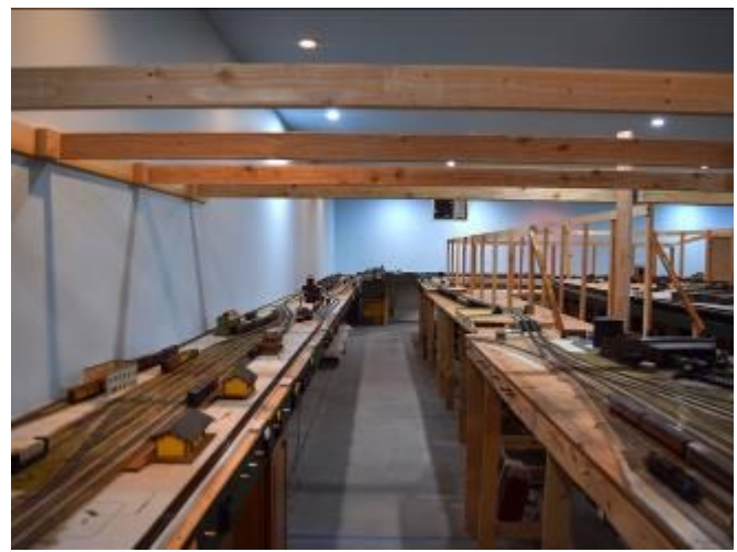
And The Rest Of The Addition Note The Upper Level Benchwork Under Construction (photo Ethan Doty)
