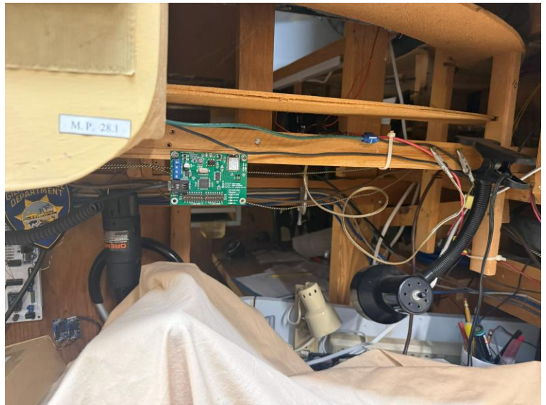
Preliminary survey says... lots of work ahead!
