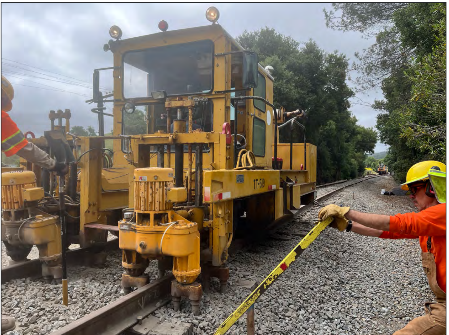
The Tamper vibrating/tamping the ballast under the rails.
