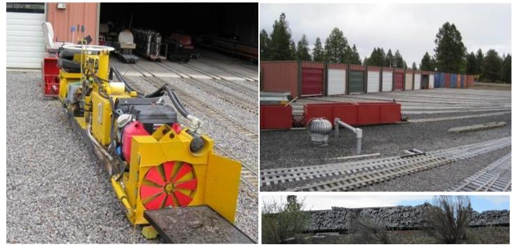
Above right: Flat cars of ties ready to be laid. Below left: Aluminum rail and wood ties are being replaced with plastic ties and steel rail (no steel rail shown here). Below right: Stacks of track panels in the yard.
