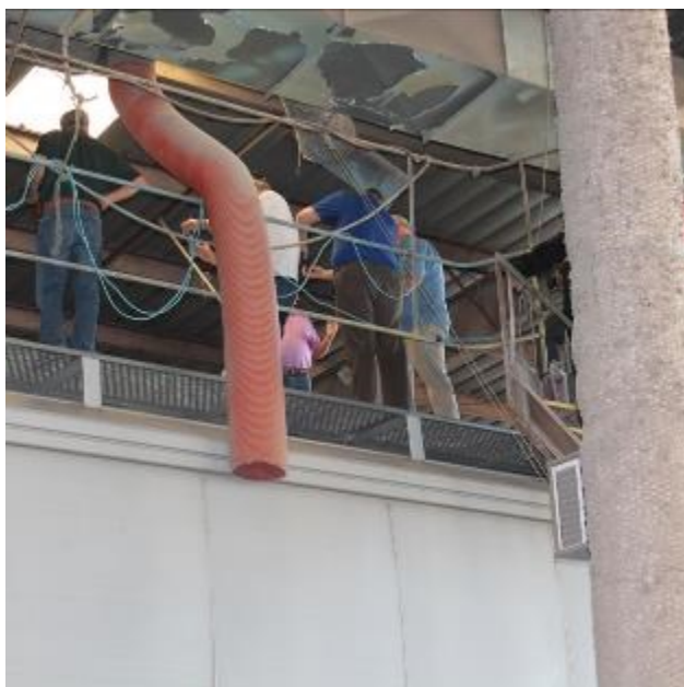
On Top of a Covered Hopper
