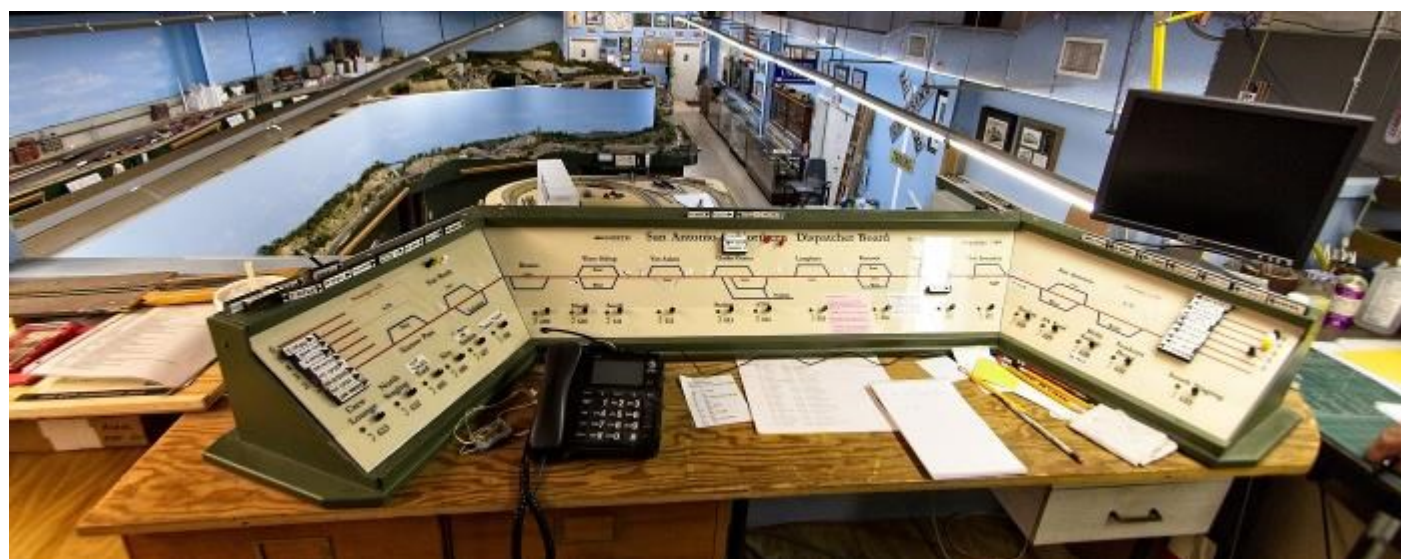
Dispatcher's desk on 2nd floor balcony.
