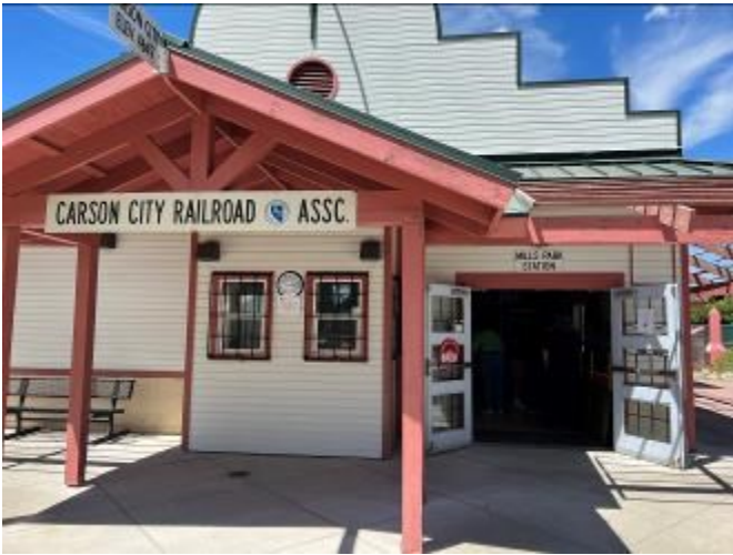
Mills Park Station (photo Lorri Meriam)
